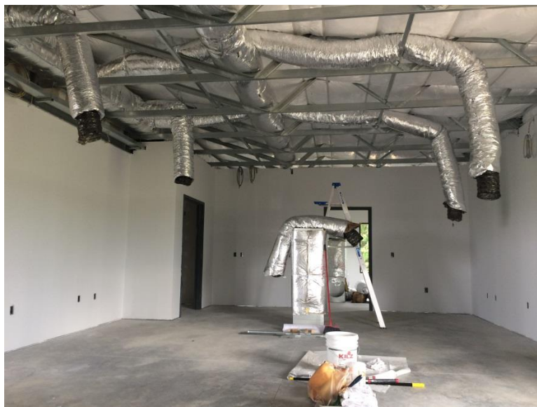
The wonderful folks at RJR Electric Heating and Air donated all the electrical, lighting and HVAC installations, putting in all the equipment and ductwork that was donated by Chisholm Service, Inc. Mickey and his crew (above left) work to squeeze all the ductwork through the roof trusses.
