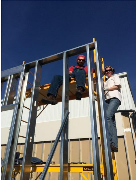
Jeremiah and Cindy (above) are up on the staging inspecting our work to ensure the framing is ready to receive their beautiful trusses.
